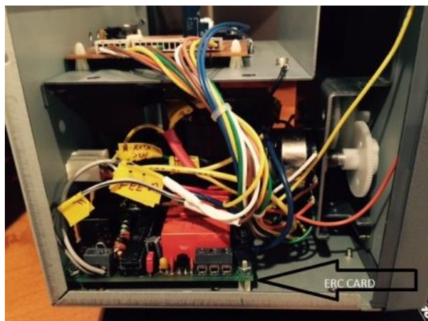
4 ERC installed in Yeasu rotator box
