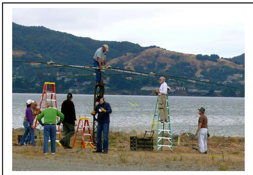
Field Day 2013 Erecting 40M beam on tower
