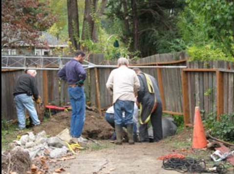
Too much old buried concrete and rock preventing a good alignment to the upstream pipe.
